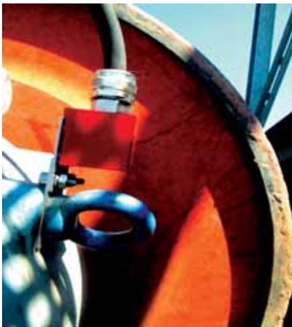
Figure 6 (a): Bearing housing temperature sensor
