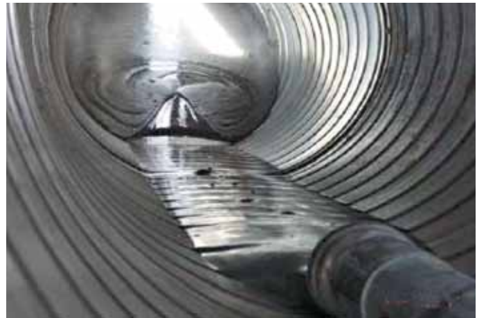
Figure 18: High strength backfill
