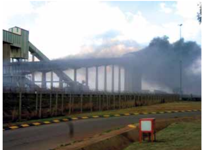
Figure 14: Surface view of conveyor fire
