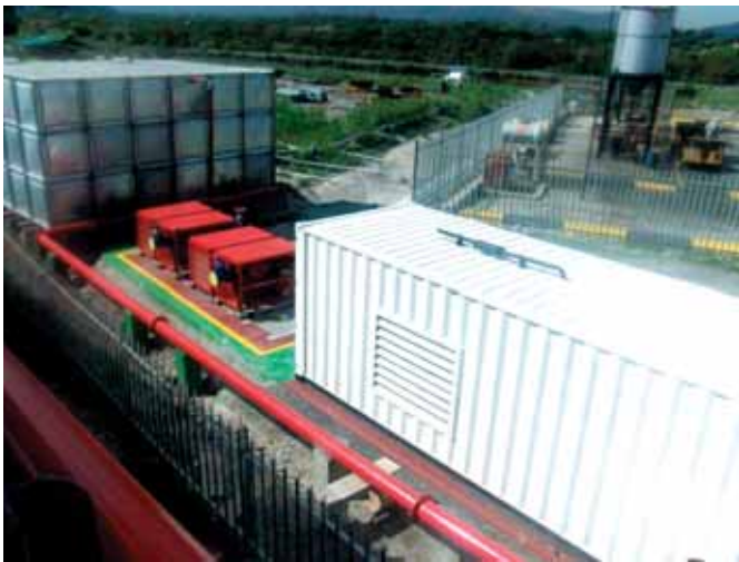
Figure 13: Surface reservoir with AFFF dosing pumps at Bathopele
