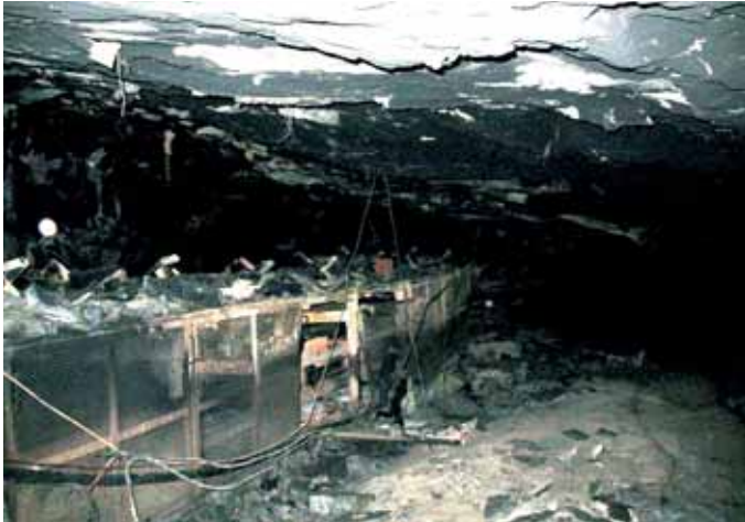
Figure 16: Damaged section of conveyor installation following fire
