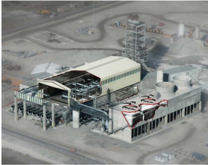
Figure - Surface refrigeration plant
